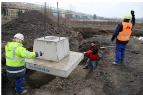
Figure 4: Precast pocket footing
