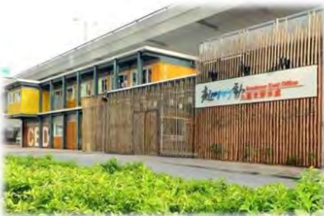
Energizing Kowloon East Office Building
