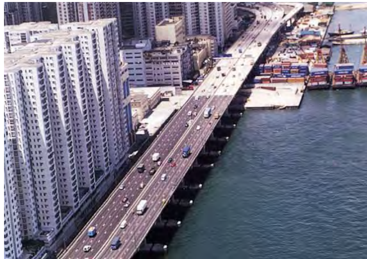
Figure 6: First PMFC trial on high speed road in Hong Kong
