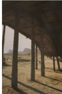
Figure 5: Internal columns (Piesik, 2012)
