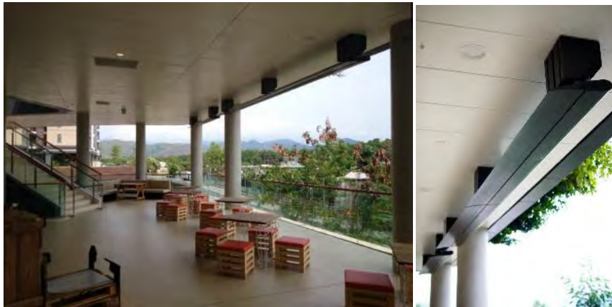
Figure 5: Installation of AIU at The Green Atrium
