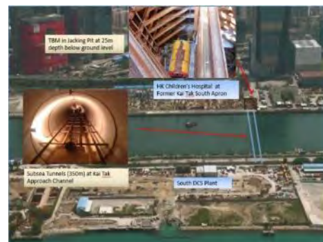
Figure 10: Two subsea tunnels (350m) constructed with TBM
