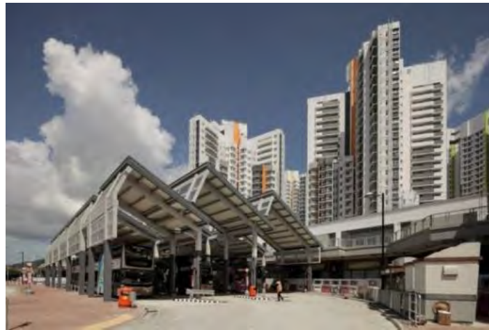
Figure 1: Special noise cover with openings for PTI at Hung Fuk Estate
