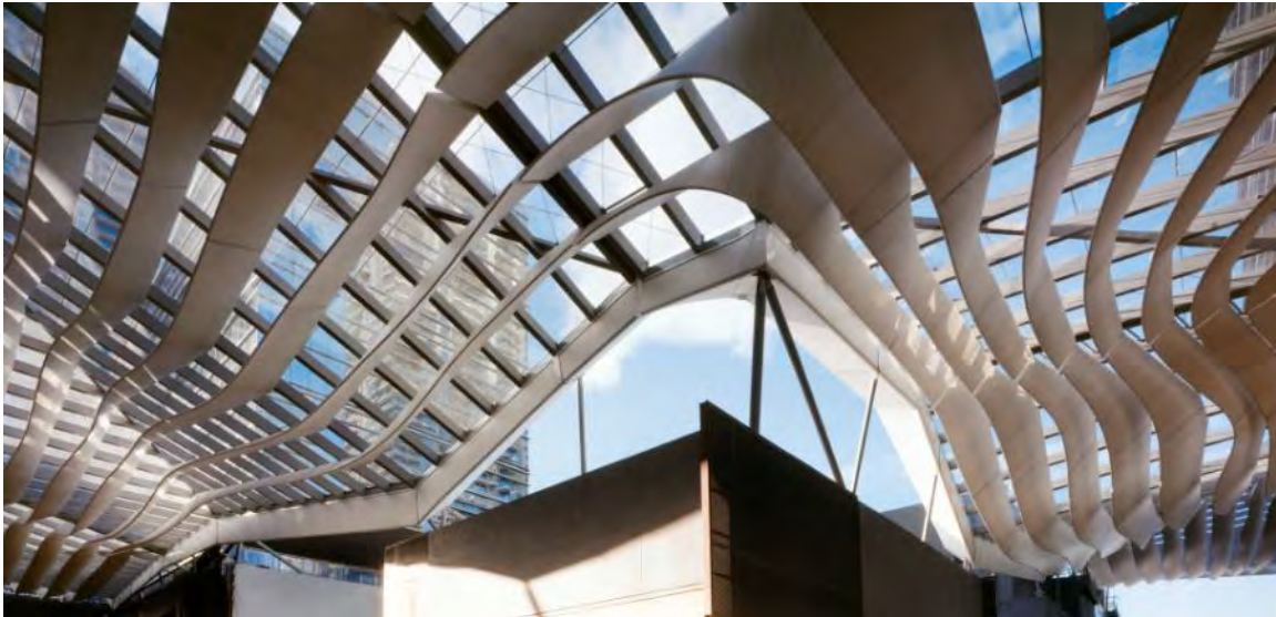
Figure 4: A 100,000 sq ft faceted canopy of steel and glass undulates between the mall, hotel, offices and residential towers
