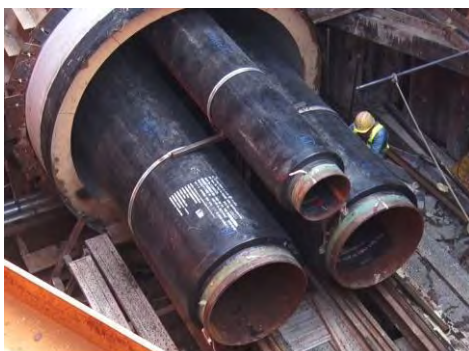
Figure 9: DCS pipes laying inside the underground tunnel
