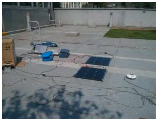
Figure 9: Outdoor test system in the 6th floor of Block Z
