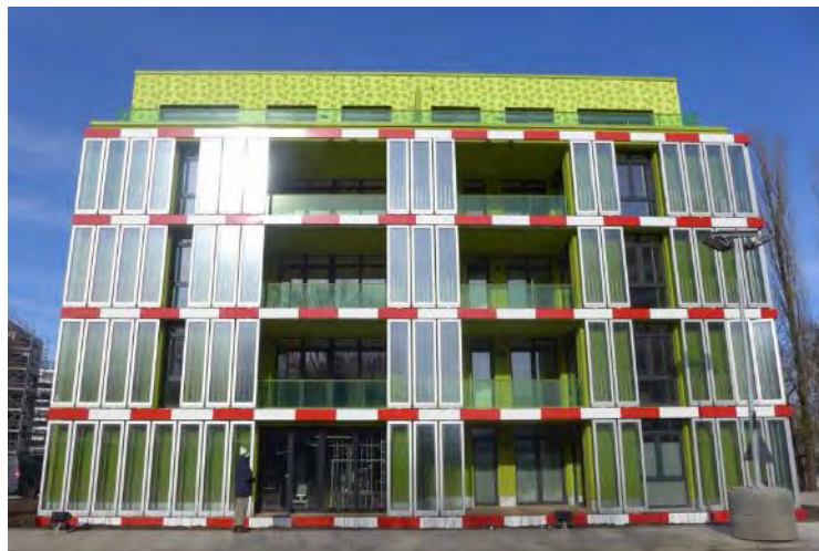
Figure 1: The BIQ is setting new standards as the first building in the world to have a bioreactor façade. Microalgae are cultivated in the glass elements that make up its "bio skin"
