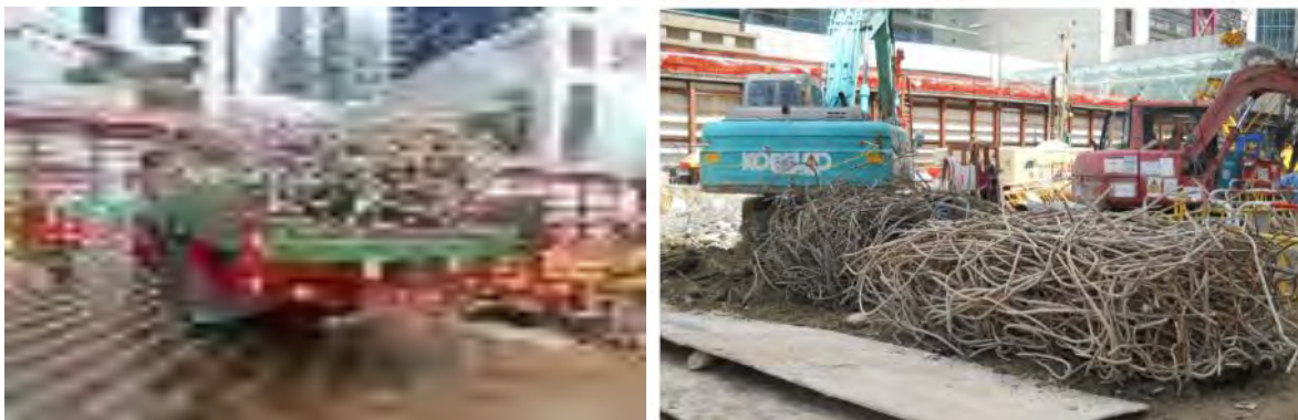
Figure 2: Recycling of waste metal in TKP2A project during demolition
