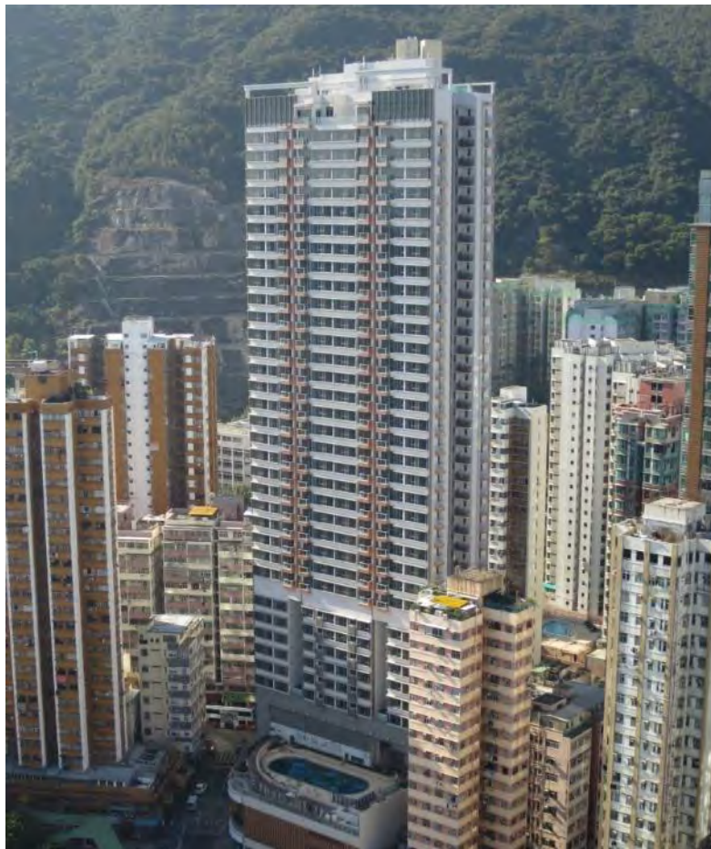
Figure 19: The generational integration design of Harmony Place comprises lower-level senior hostel for lease, and higher-level private residential units for sale.
