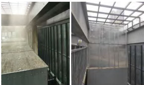
Figure 6: Cooling tower exhaust before and after retrofitting
