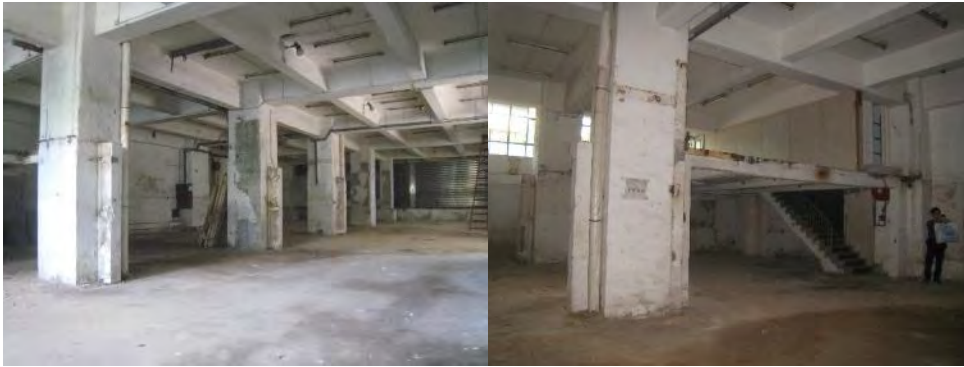
Figure 2: Space vacated waiting for demolition
