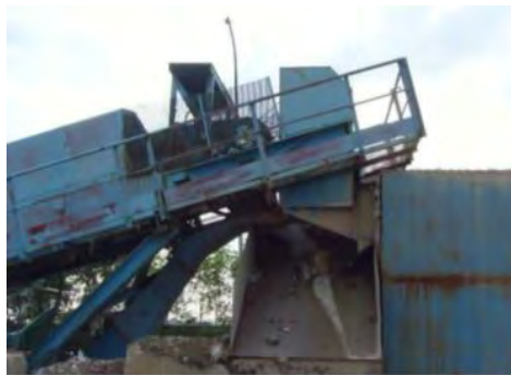
Figure 5: Wind-blower for sorting light weighted unwanted constituents in C&D Waste at the sorting facility in Tseung Kwan O Area 137
