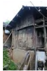
Figure 9: The gable structure
