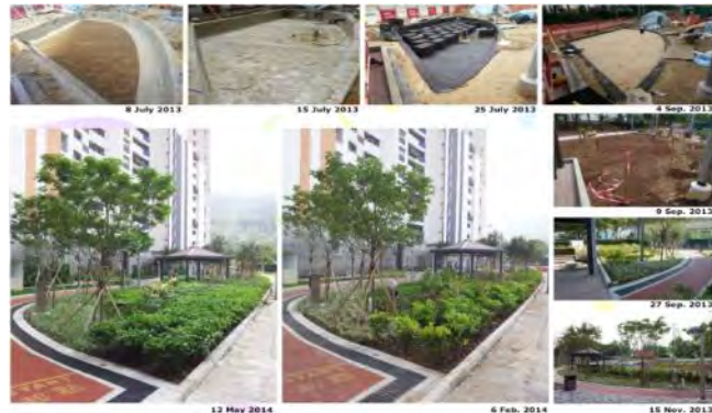
Figure 7: Construction of ZIS at trial planter
