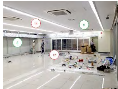
Photo 2: Designed technologies, the interior
