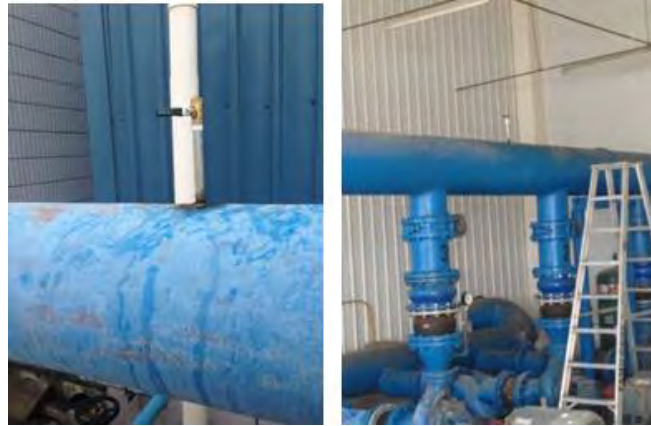
Figure 2.3b: Vent valves installed
