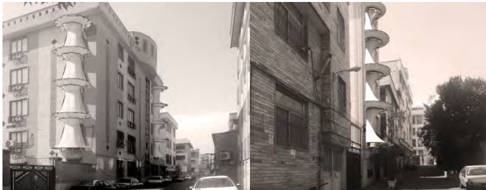
Figure 8: The proposed adaptive wind-catcher concept in the existing urban context of Tehran
