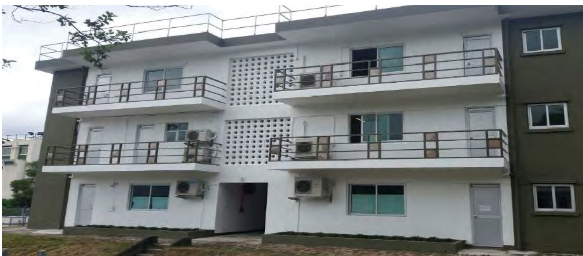
Figure 5: The latest view of the renovated buildings.
