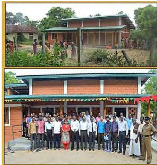
Figure 4: One of the completed community center building made out of Mud: Concrete Blocks in Batticaloa
