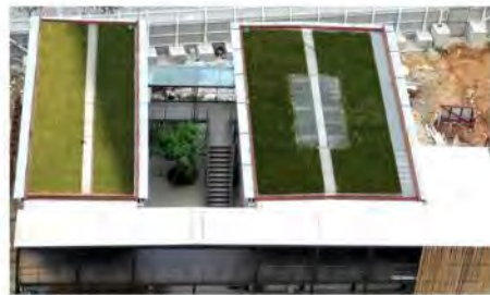
Roof greening (Fig. 5)
