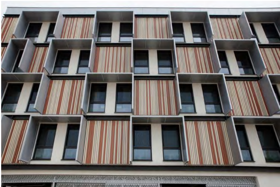
Figure 6: The passive house hotel, innovative neopor® insulation, efficient spray foam insulation for the roof (Source: BASF)
