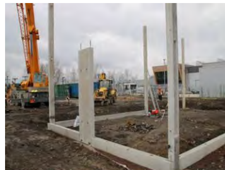
Figure 5: Assembling of subtle columns, stiffening wall and foundation sills
