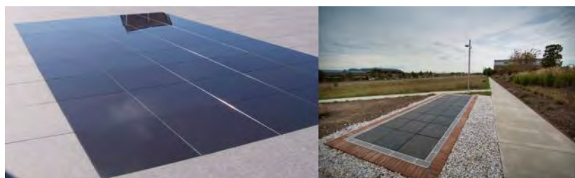
Figure 3: A walkable PV pavement system
