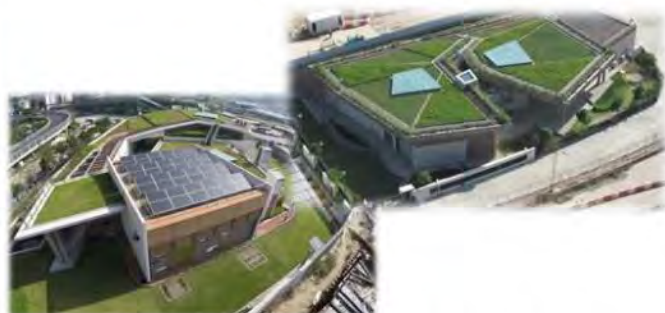
Kowloon City No.1 and No.2 Sewage Pumping Stations
