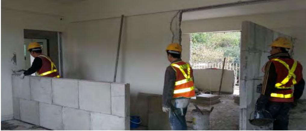
Figure 9: Construction of partition walls with recycled chemical gypsum
