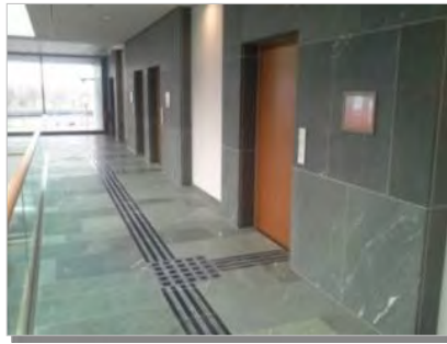
Figure 11: Tactile guidance strips
