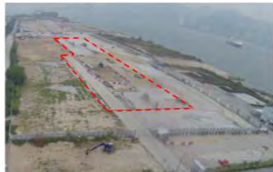
Figure 5: The South Plant located at the underground of Ex-runway of Kai Tak Airport.
