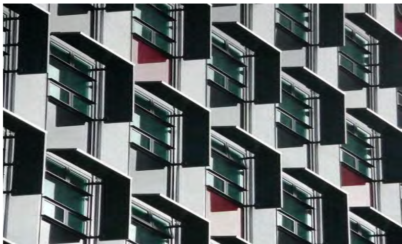
Figure 1: The East view showing the operable windows and overhangs used as solar shading
