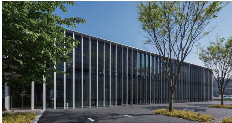
Figure 1: Exterior of the building after renovation
