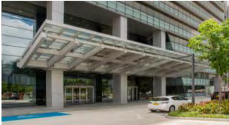
Building integrated photovoltaic panels in canopy
