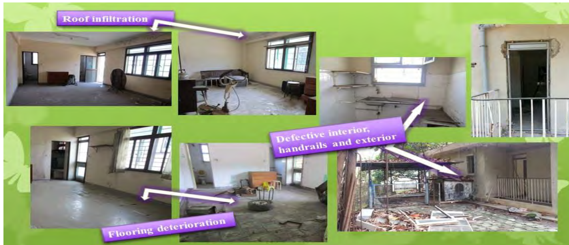
Figure 2: The condition of Sheung Shui Staff Quarters before renovation.
