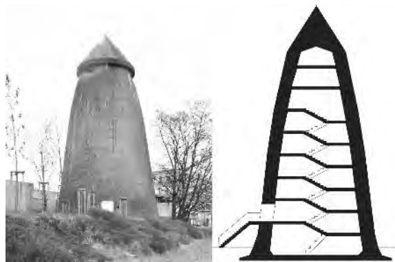
Figure 1: Outside view [source: author] and section of a variant "winkel" bunker [source: 11]
