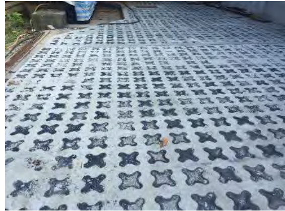
Figure 5: Grasscrete under Construction (2)
