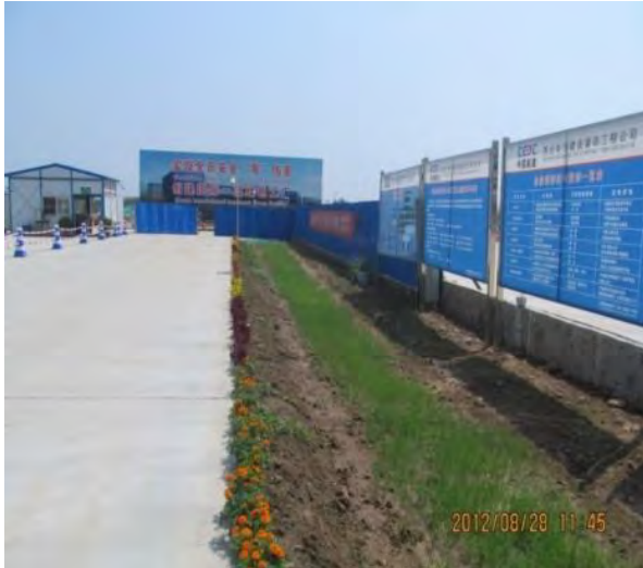
Figure 4: Temporary plant and waterway
