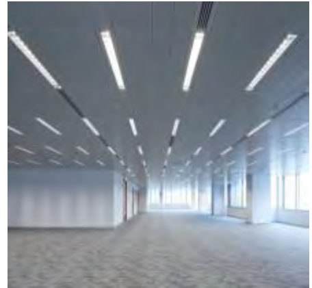
LED lighting at part of the office areas
