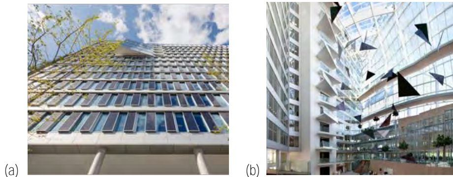
Figure 6: (a) BIPV on the South Façade of the 'Edge' (Source: Ossip van Duivenbode); (b) Fifteen-Storey North-Facing Entrance Atrium (Source: Raimond Wouda).
