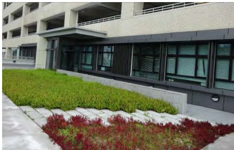
New green roof
