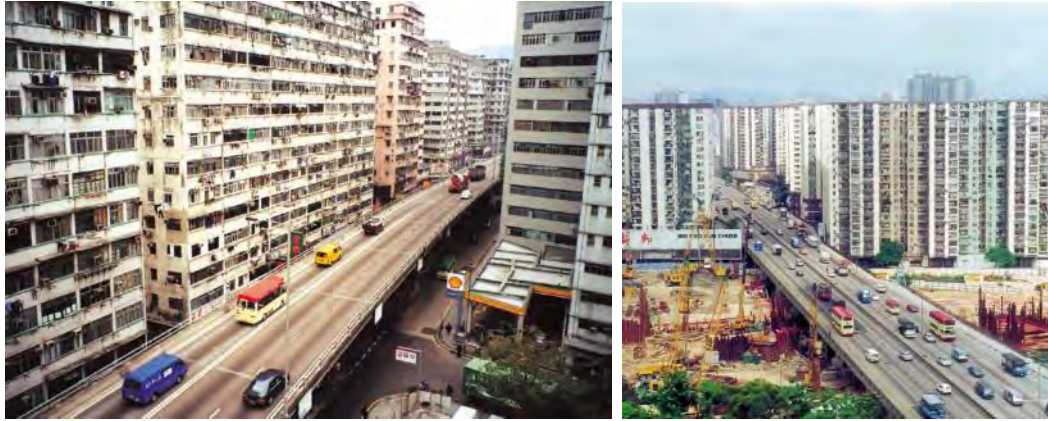
Figure 1: Trunk roads built right next to residential blocks in the 1980s
