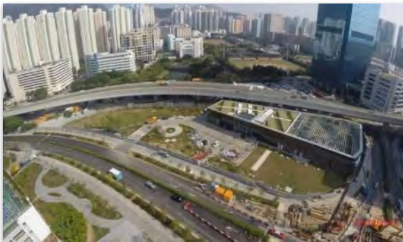
Figure 4: The North Plant located at Shing Kai Road
