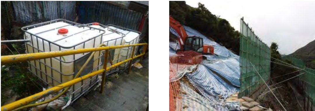
Figure 5: Water pollution control measures (left photo) and air pollution control measures (right photo) for the LPMit works
