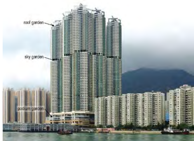
Figure 1: Podium garden, sky garden and roof garden at a residential development in Hong Kong.
