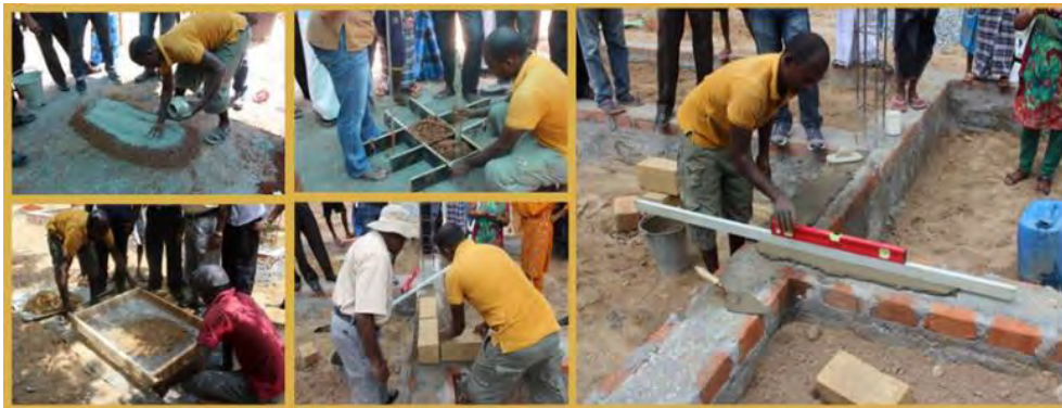
Figure 2: Educating the community people through the building process
