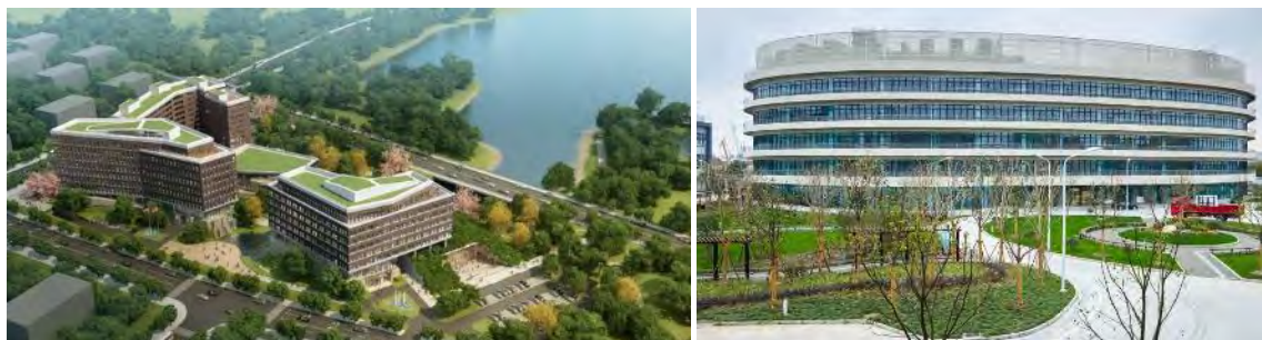
Figure 5: The German Enterprise Centre, Qingdao, DGNB Pre-certificate, Source: Sino-German Ecopark Real Estate AND BASF R&D Center Shanghai, DGNB Certificate, Source: BASF
