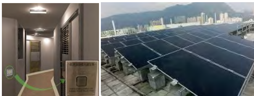
Figure 2: Two-level lighting control system (normal mode: 50 lux; triggered mode: 85 lux) (left); Roof photovoltaic system in a public housing development in 2010s (right)
