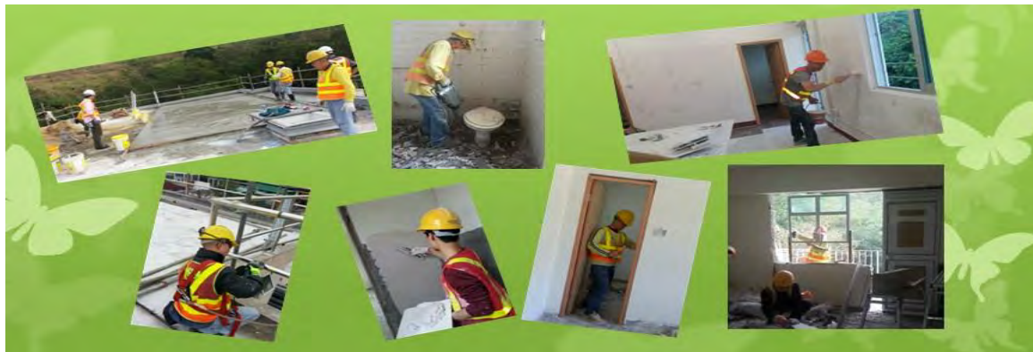
Figure 3: Scope of renovation works of Sheung Shui Staff Quarters.
