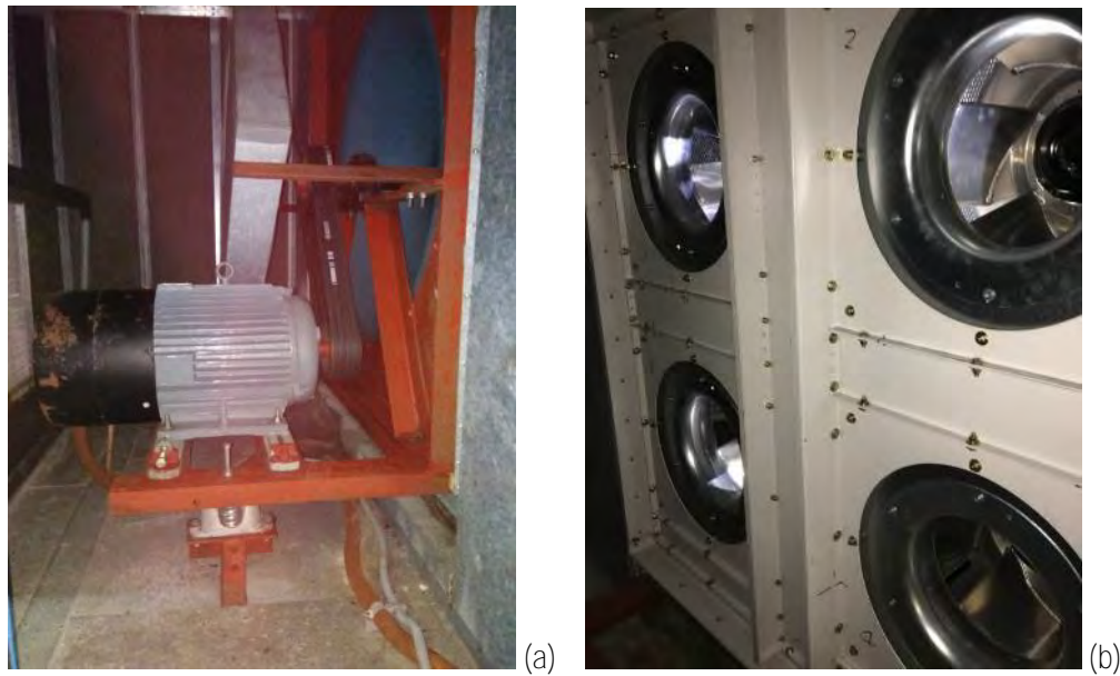
Figure 1: (a) Belt driven fan and (b) EC motor plug fan
