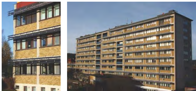
Figure 2: Sollefteå hospital with the energy producing solar shading.
