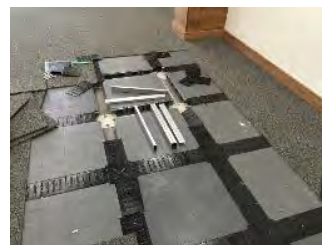
Raised floor system and carpet were made of recycled materials
