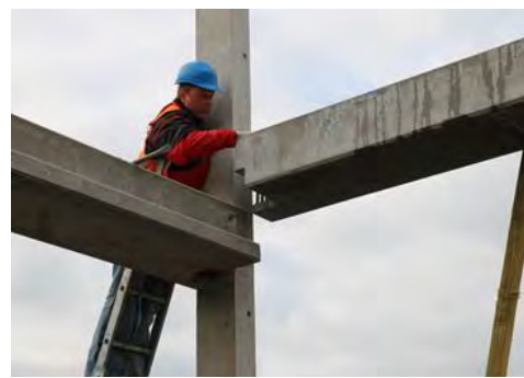
Figure 7: Assembling of transverse bracing on girder fitted on Peikko's corbel
