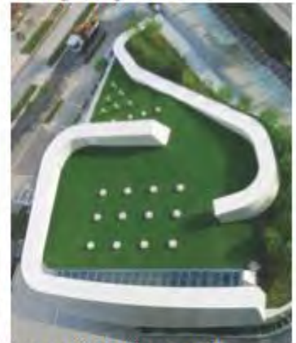
Community hall green roof
