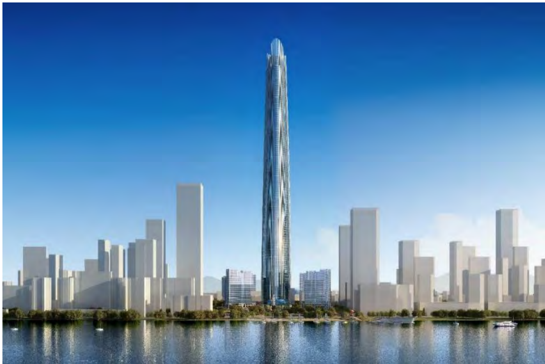
Figure 4: Wuhan CTF Finance Centre: Visually connecting and physically integrating with the community
