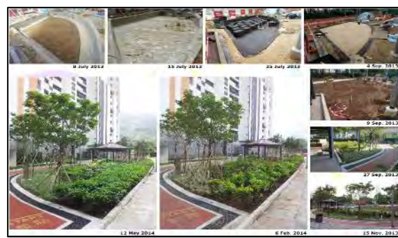
Figure 2: Construction of ZIS at trial planter
