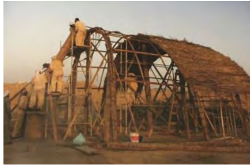
Figure 112: The vault during construction (Piesik,2012)
