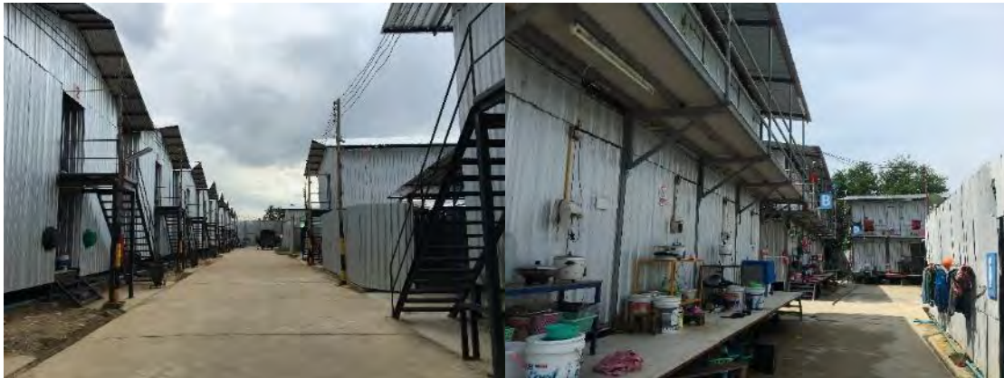
Figure 2: L.P.N. construction camp
