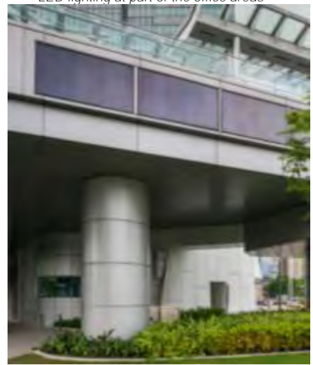
Solar hot water panel in external landscaped area
